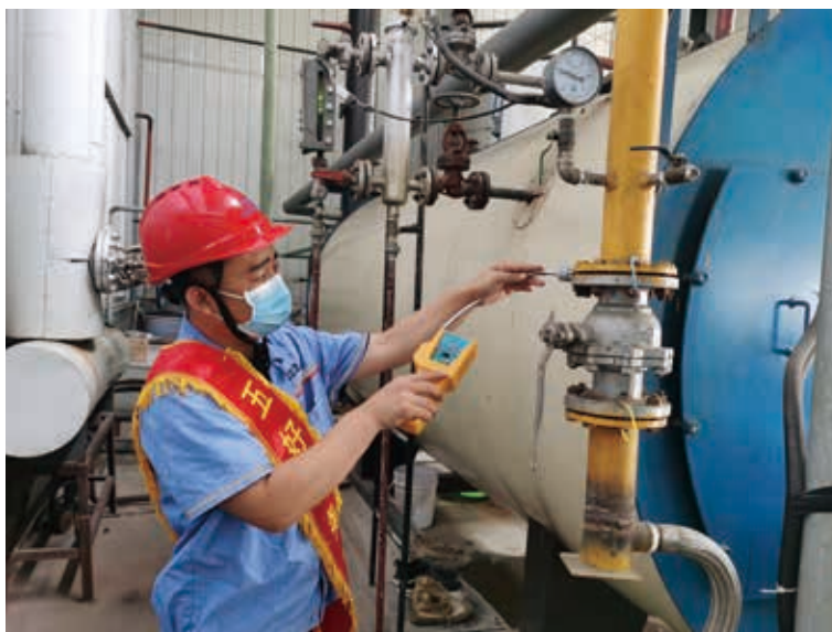
Safety examination by Tangshan Subsidiary Company 唐山公司安全檢修
